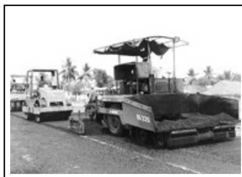
Paver Finisher with Sensor in operation for construction of NH- 9 over 48 KM from Nandigama to Vijayawada in Andhra Pradesh for NHAI
