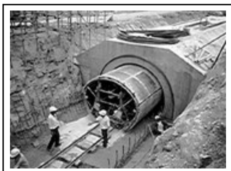
Upper Dam Diversion Culvert Works for Purulia Pumped Storage Project for Taisei Corporation
