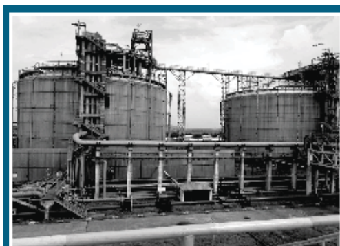
Cryogenic LPG Storage Tank at BPCL Uran
