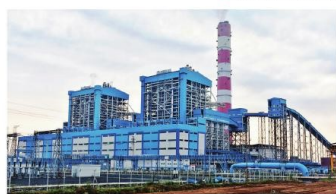
• Main Power House Unit I & amp; II at NTPC Ltd 2x800 MW Super Thermal Power Project at Gadwarwa (2013-20)
