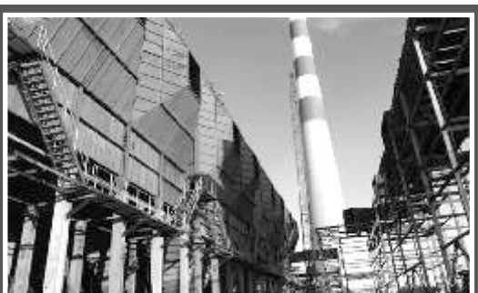
Erection, Testing, Commissioning of ESP, Boiler, and other Auxiliaries at Sagardighi, W.B. for M/s BHEL
