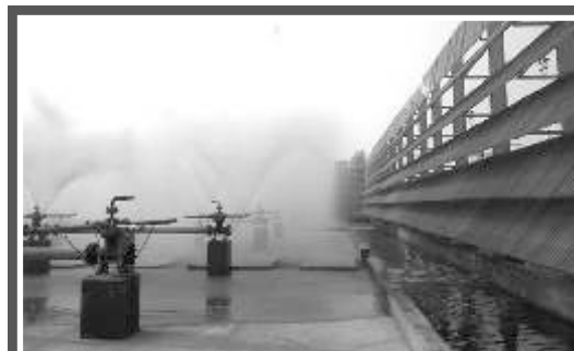
Turnkey execution of Mist Cooling Water System for Gas Cracker Unit at GAIL, Pata
