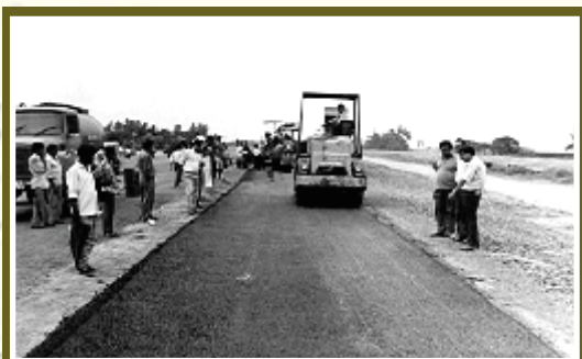
Two Lane Expressway with Service Roads at Dankuni for PWD, West Bengal
