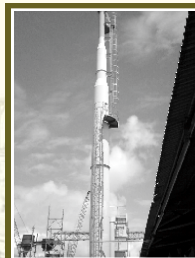
Stack at Captive Power Plant for NALCO, Angul
