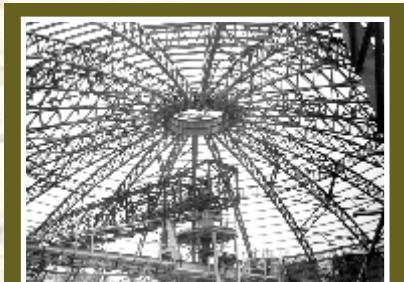
Construction of Blending Silo at Cement Plant for Penden Cement Authority Ltd. at Gomtu, Bhutan
