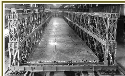
Manufacture of Bailey Type Unit Bridge at Howrah Workshop
