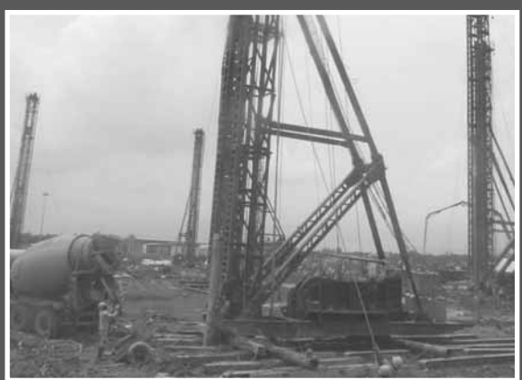
Power Plant of Haldia Energy Ltd.
