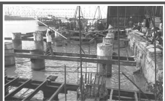
Hooghly River Front Development Work of Kolkata Municipal Corporation
