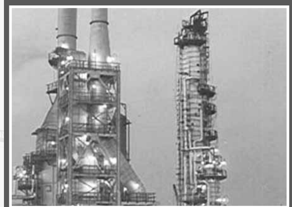
VDU Furnace at IOCL, Haldia
