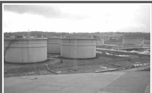
Tankage Work at MRPL, Mangalore
