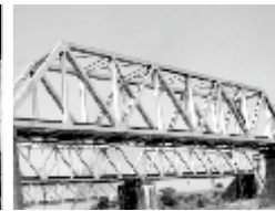
Rail & Road Bridges
