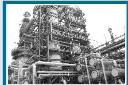
Piping and equipment work of NHT / CCR Unit at Visakh Refinery, HPCL
