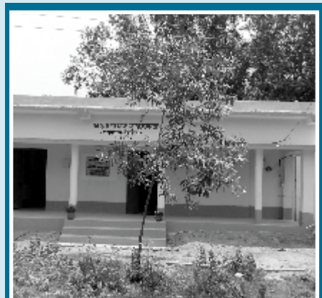
Construction of two room Health Centre including toilet for Kuchia Bhalo Pahar at Purulia district, W.B. under Swachh Bharat
