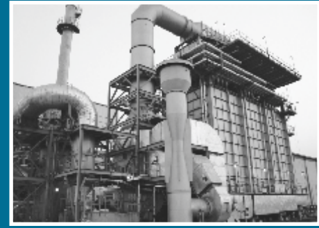
Radiant Heater at MCPI, Haldia
