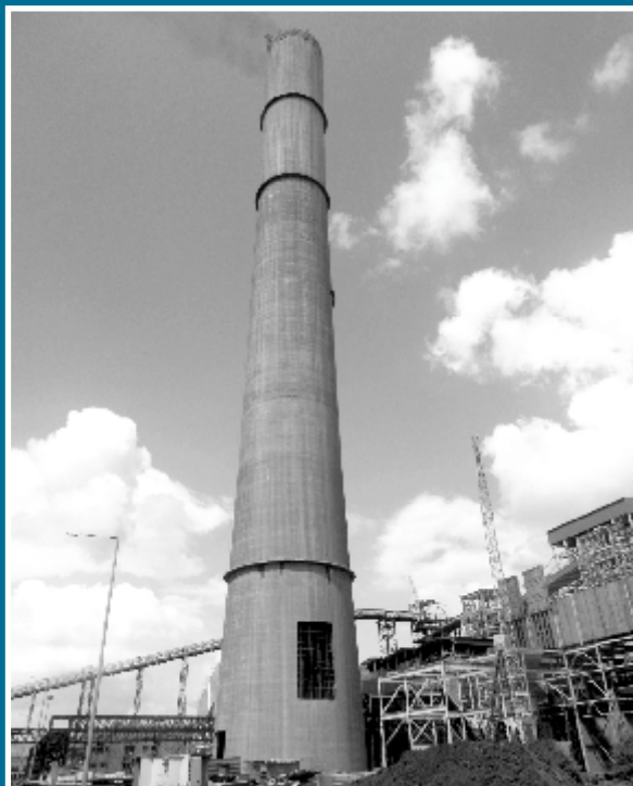
Twin Flue Chimney of height 275m at Gadawara, MP for M/s. NTPC
