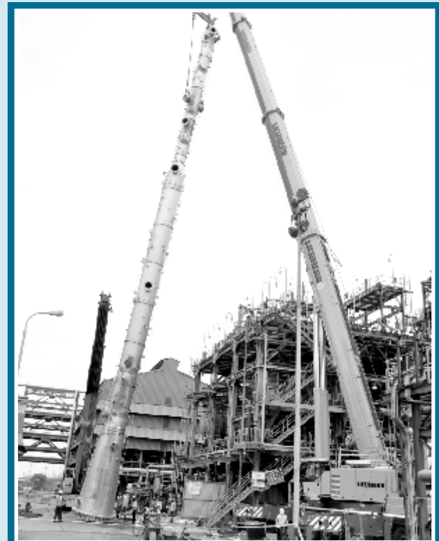
Column erection work at Visakh Refinery, HPCL
