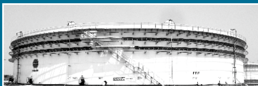
Crude Oil Storage Tank at IOCL, Paradip
