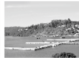
Piling & Marine Work
