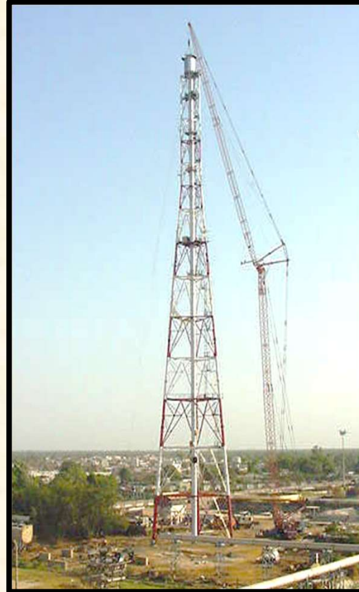
Erection of Flare Tip during Flare Stack Package on EPC Basis at IOCL Gujarat Refinery
