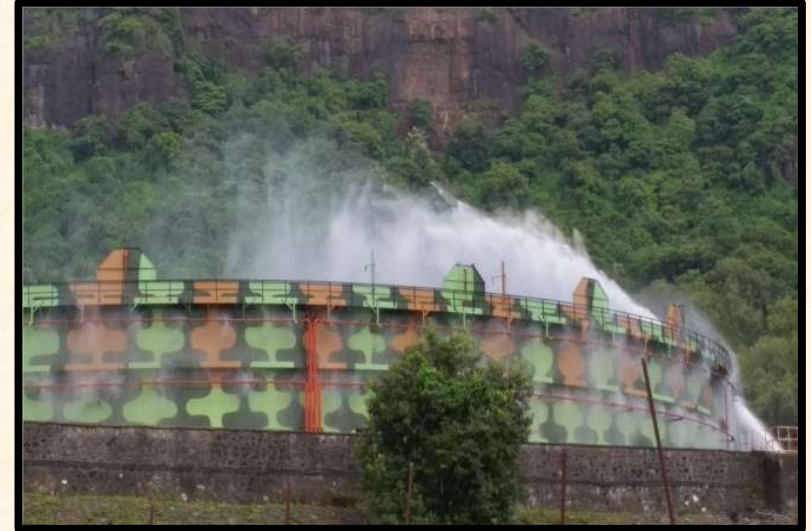
Fire fighting system for Crude Oil Storage Tanks at ONGC, Uran.
