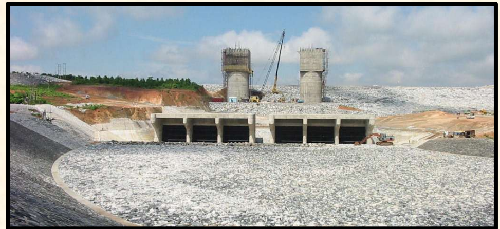
Power Intake Area and Gate Shafts
