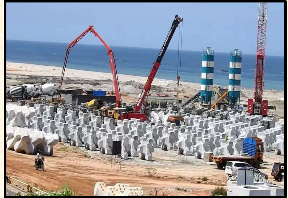
Casting and Staking of Accoropodes for break water development of Vizhinjam Port at Kerala of Vizhinjam International Seaport Ltd. For Adani Group
