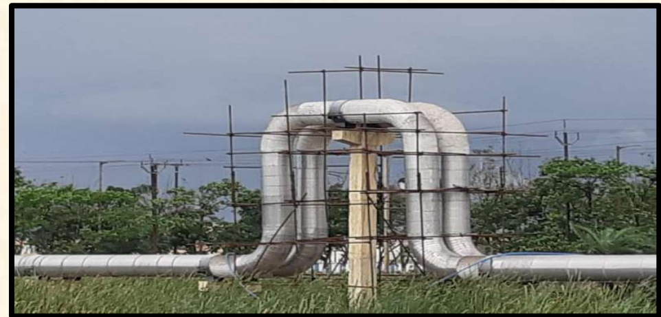
Propane and Butane pipeline Double Wall 18"/25" size Cross-Country Pipeline for BPCL Haldia
