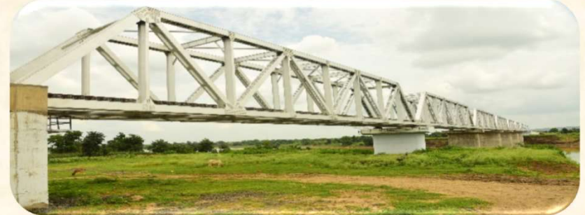
Fabrication and Launching of open web through girders for major bridges between Jhalawar-Aklara section for W.C.
