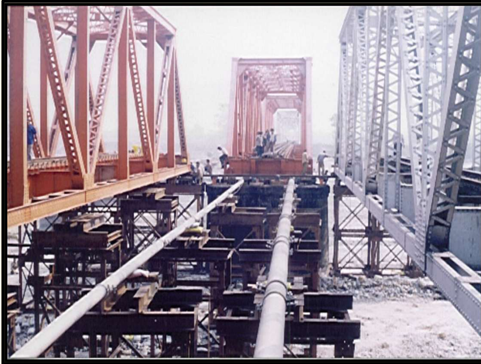
Regirdering of 7 spans X 45.70 metre each of Diana Bridge for Northeast Frontier Railway
