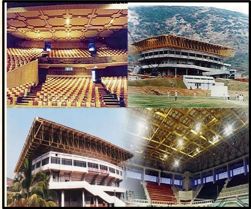
Planning, Design, Detail Engg. & Construction of Sports & Cultural Complex at Salagramapuram for Visakhapatnam Port Trust
