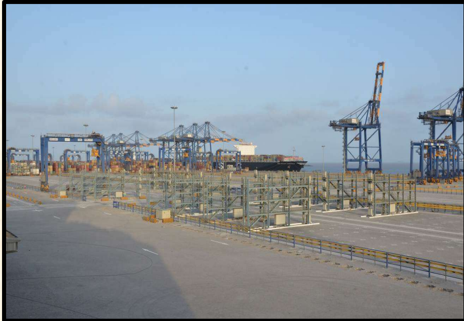
Backup Yard at Adani Mundra Port, Gujarat
