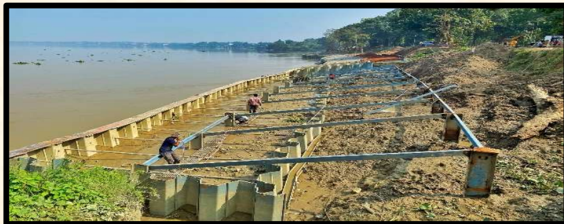
Sheet Pile & ISMB Driving
