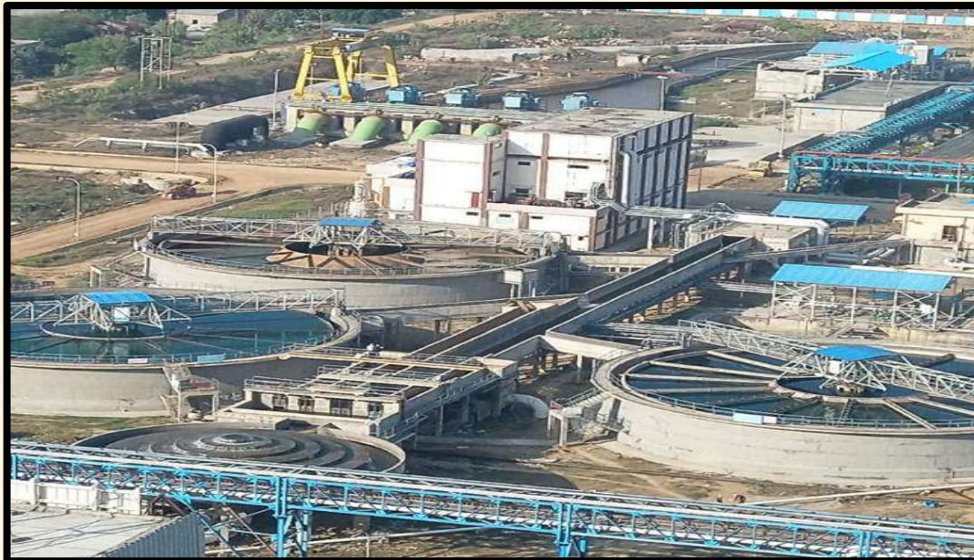
Water Pre Treatment and Liquid Effluent Treatment Plant at MUNPL Meja, Allahabad on EPC basis
