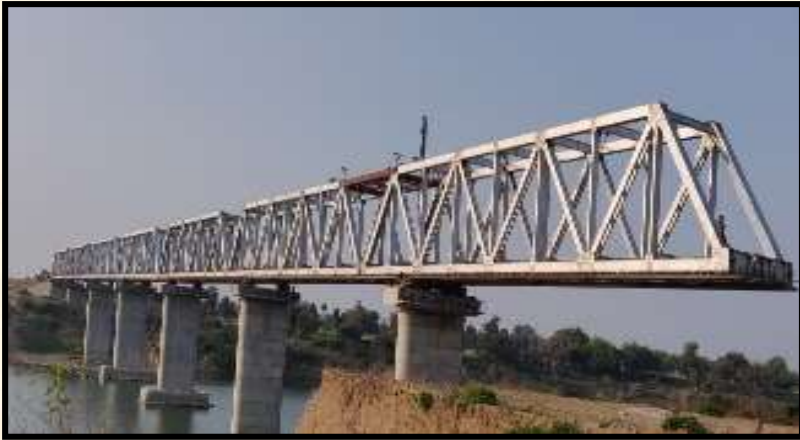
Railway Bridge at Kota for West Central Railway
