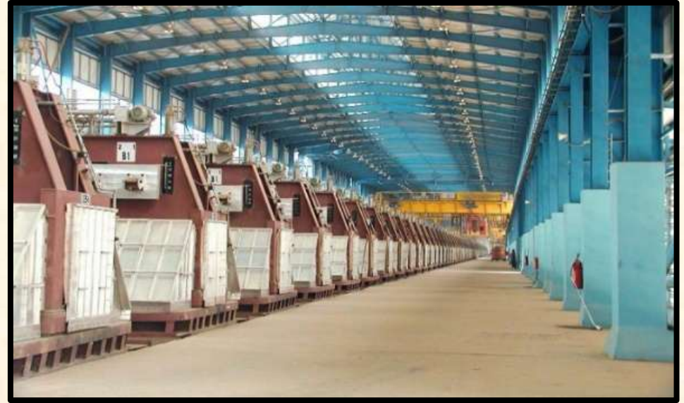
Pots Supporting Beams & other associated parts at Bharat Aluminium Co. Ltd, Korba
