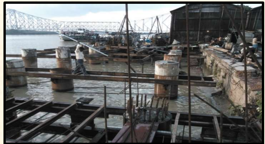
Hooghly River Front Development Work of Kolkata Municipal Corpn.
