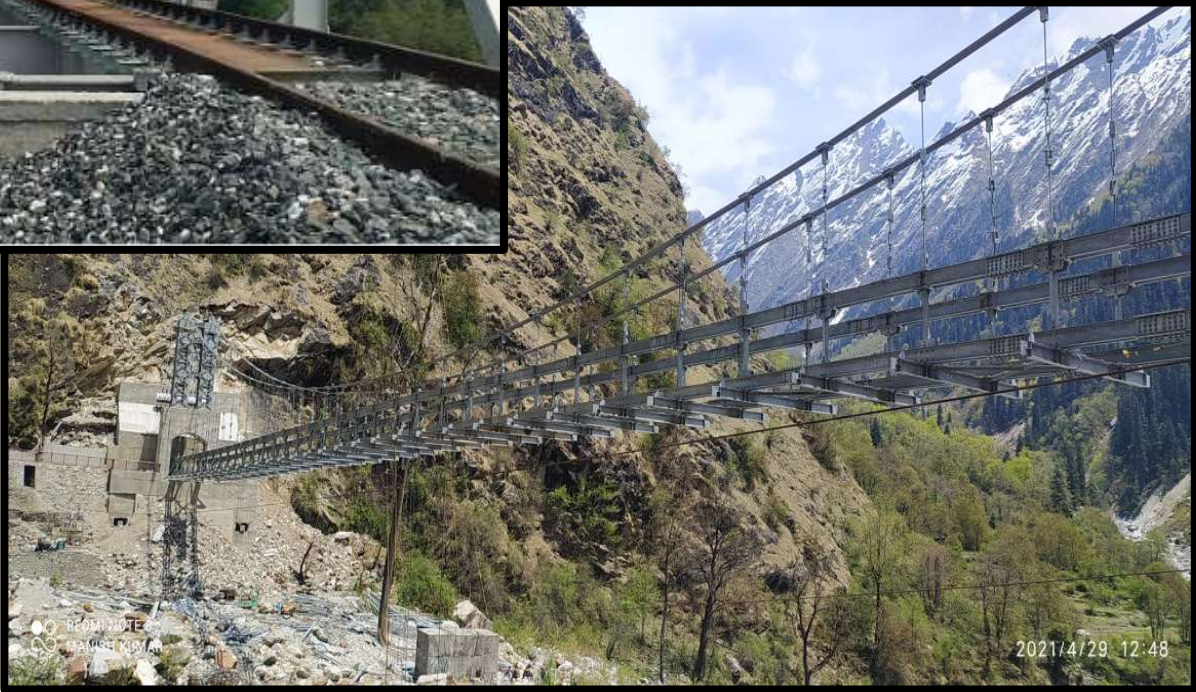
135 Mtr span Suspension Pedestrian Steel Bridge on Govindghat to Ghangharia Road at KM 10 in Chamoli District for PWD, Uttarakhand on PMC Basis
