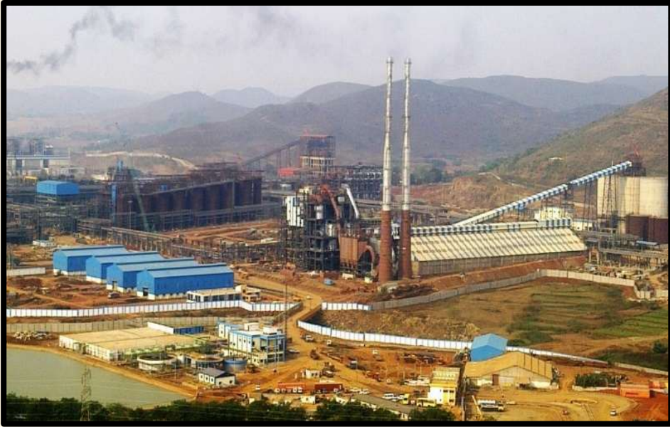
Rayagada Alumina Refinery Project of Aditya Birla Group
