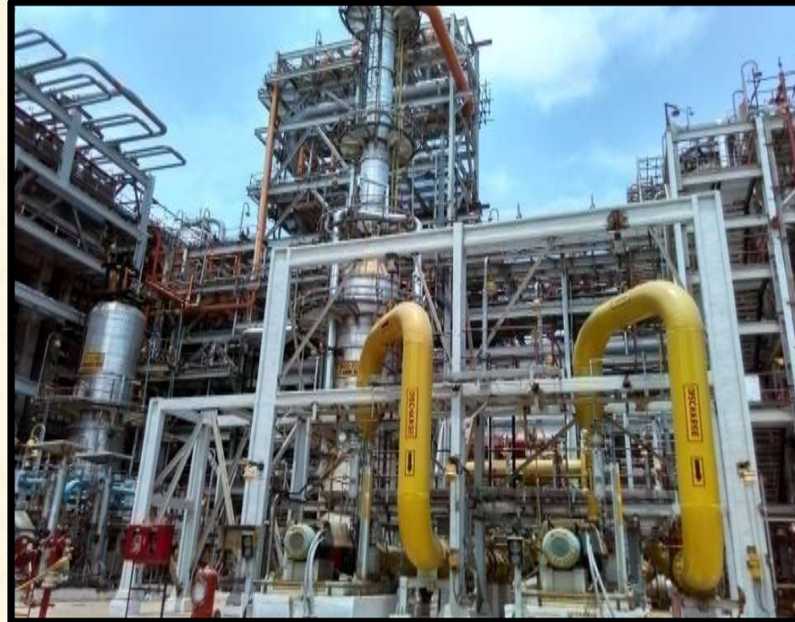
Unit Piping Work at IOCL Paradip Refinery Project
