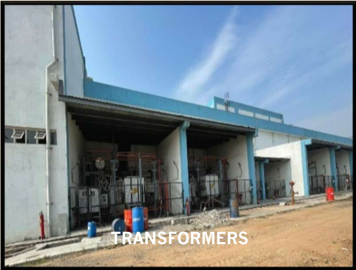
Electrical and Instrumentation Work at IOCL Vadodara
