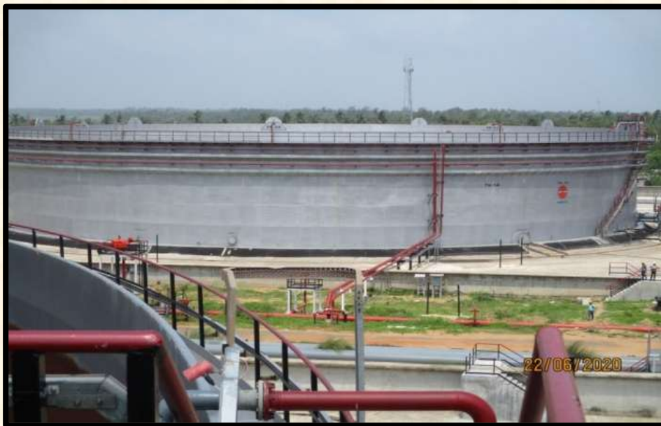
79 M Dia Double Deck Floating Roofs at IOCL Paradip Refinery on EPC basis
