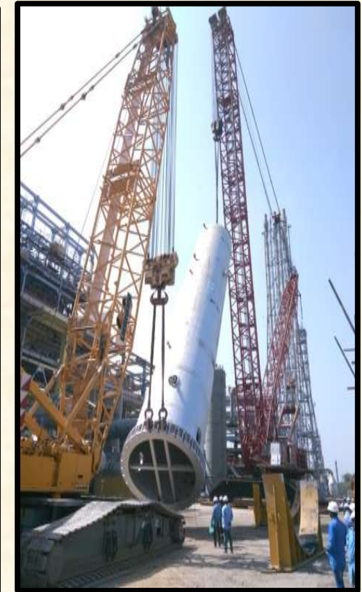
Heavy equipment erection at BPCL Mahul
