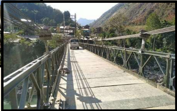
400 ft. Span Bailey Suspension Bridge over over River Kamla at Tamen for Arunachal Pradesh PWD
