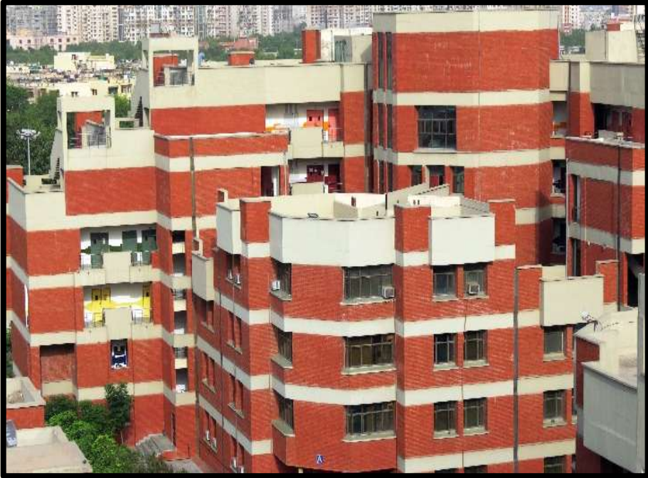
Construction of Administrative Block (G-3), Library Blocks, Academic Blocks at Guru Govind Singh Indrapastha University, Delhi
