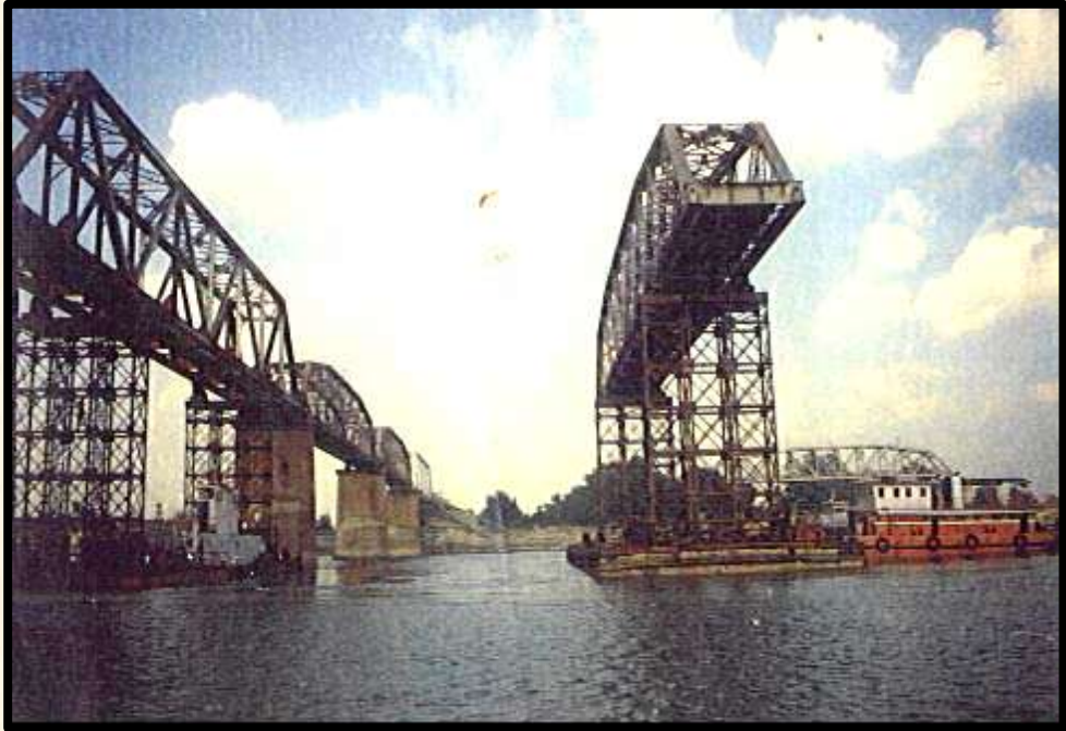
Regirdering of Railway Bridge at Majhi Ghat, Bihar for Northeast Frontier Railway
