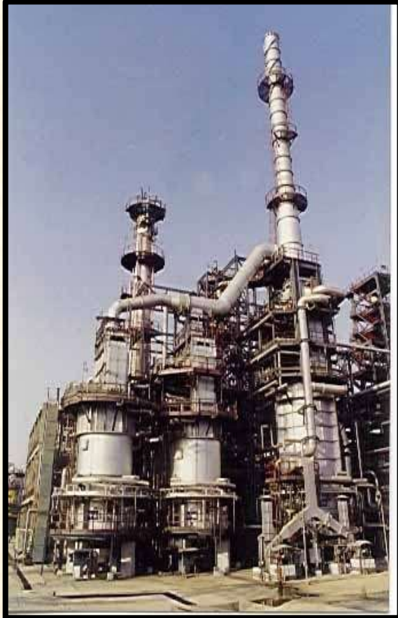
Construction of 3 Nos. Non-IFP Heater in Panipat Refinery Project of IOCL
