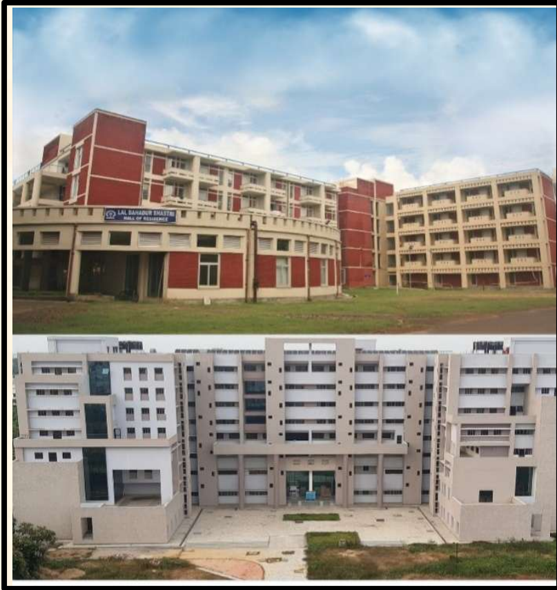
Buildings, Hostels, Residential quarters and other Infrastructure at Indian Institute of Technology, Kharagpur on PMC Basis
