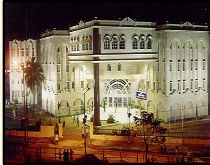
Construction of West Bengal National University of Juridical Sciences at Salt Lake City, Kolkata
