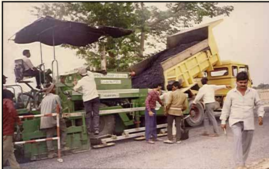
Sonauli-Gorakhpur Road Project for UP-PWD (Under Loan Assistance from World Bank)
