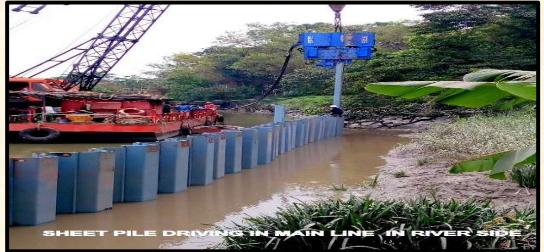
Sheet Pile Driving of Main Line of river side
