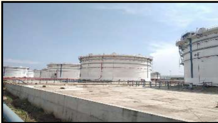
Storage tanks for oil companies
