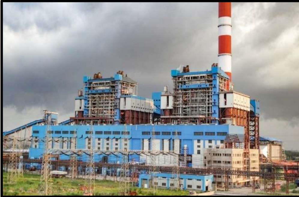
Power Block Unit for 2X500 MW Unit # 1 & 2 at Durgapur Steel Thermal Power Station of DVC at Andal Unit-3
