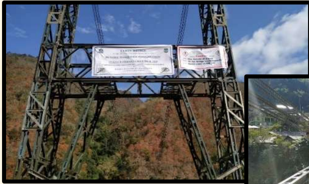
Supply, Fabrication and Erection of world's longest Bailey Bridge of 1400 ft. span, 'Col. Chewang Rinchen Setu', for Border Roads Organisation, strategically located on Shyok River between Leh and Karakoram Pass.
