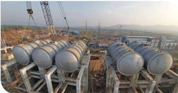
Catofin Reactors at GAIL USAR PDH-PP.
