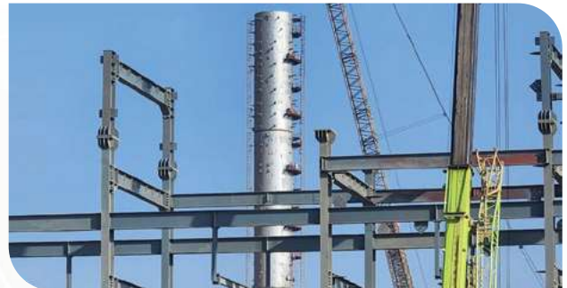
Product Splitter column of Wgt.1600MT
