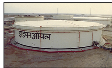
Cone Roof Tank at Kandla F.S.T. for IOCL
