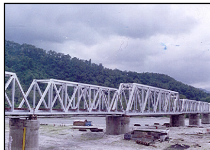
Regirdering Work in progress over River Diana For N.F. Railway
