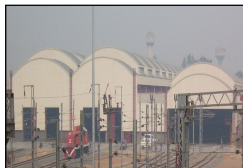
Workshop at Khyber Pass Depot of Delhi Metro Railway Corporation
