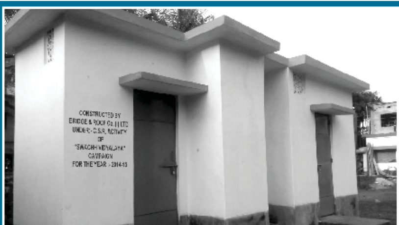
Construction of Toilet Blocks under Swachh Bharat Abhiyaan at North Dinajpur, West Bengal
