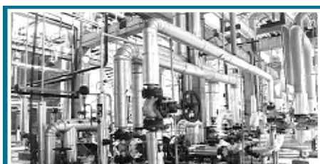
Piping Work at LLDPE of IOCL, Panipat
