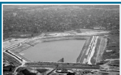
Ash Disposal Pond at Durgapur Steel TPP of DVC
