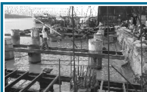
Hooghly River Front Development Work for Kolkata Municipal Corporation
