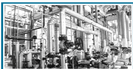
Piping Work at LLDPE of IOCL, Panipat
