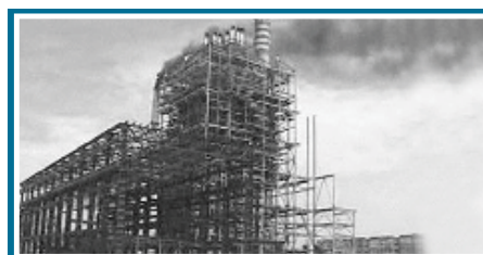
Structural Steelwork at Sanjay Gandhi TPP at BHEL, Birsinghpur
