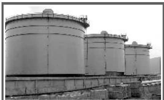
White Oil Terminal at HPCL Vizag
