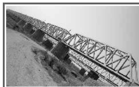
Riveted Steel Girder Bridge at Bilaspur for S.E. Railway
