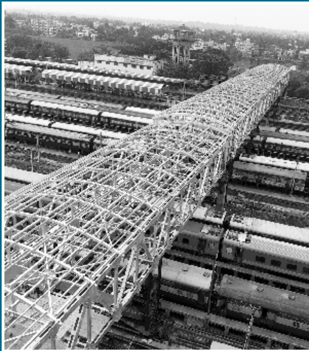
162m long Foot Over Bridge at Santragachi Station for South Eastern Railway
