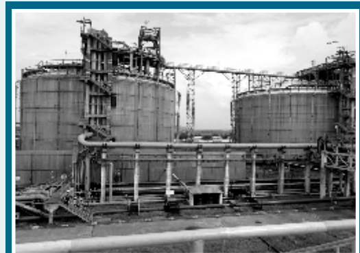
Cryogenic LPG Storage Tank at BPCL Uran
