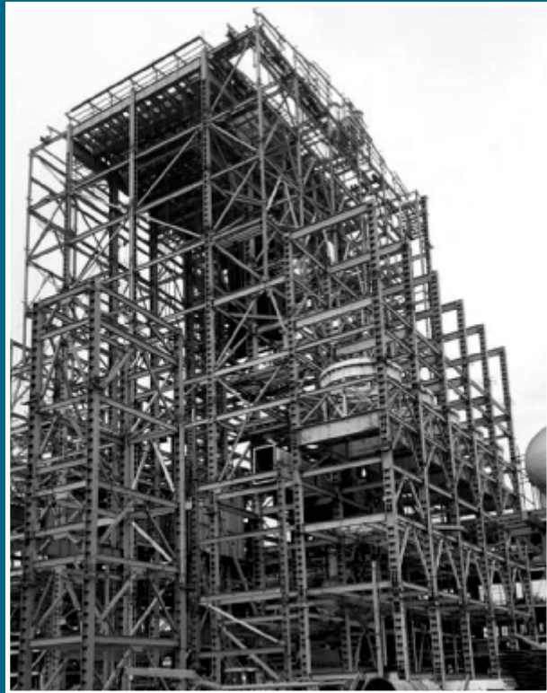
Erection, Testing & Commissioning of Boiler and its Auxiliaries for 2 X 800 MW Ramagundam Project of NTPC
