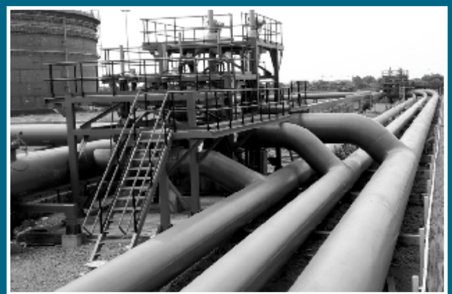
Mechanical Work at BORL Bina Terminal
