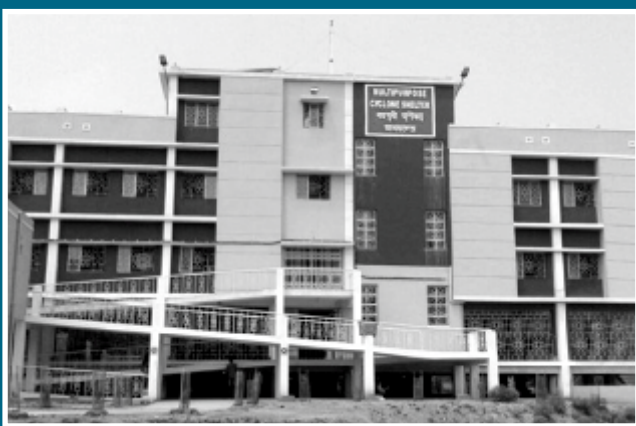
Construction on Multipurpose Cyclone Shelter under NCRMP-II at various coastal areas of West Bengal
