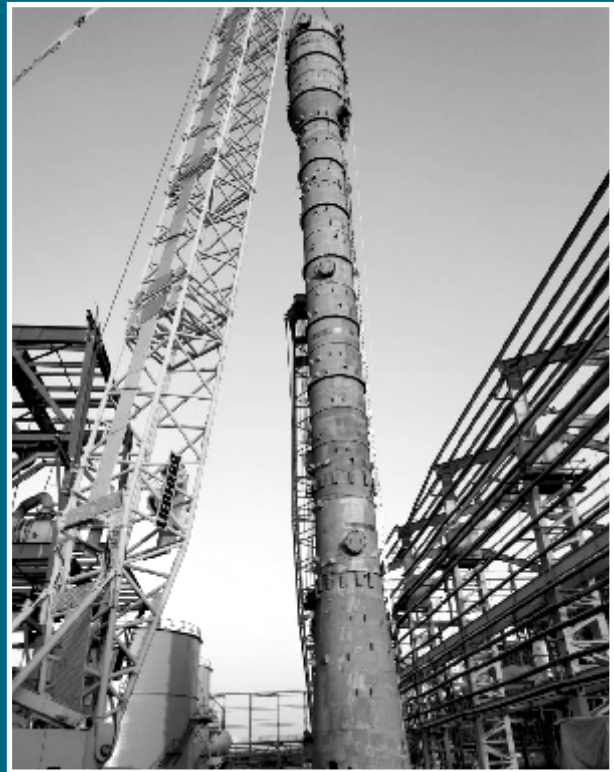
Single Stage Sour Water Stripper Column Erection, 94MT, 44m long & 2.4m dia at IOCL Haldia BS-VI Project
