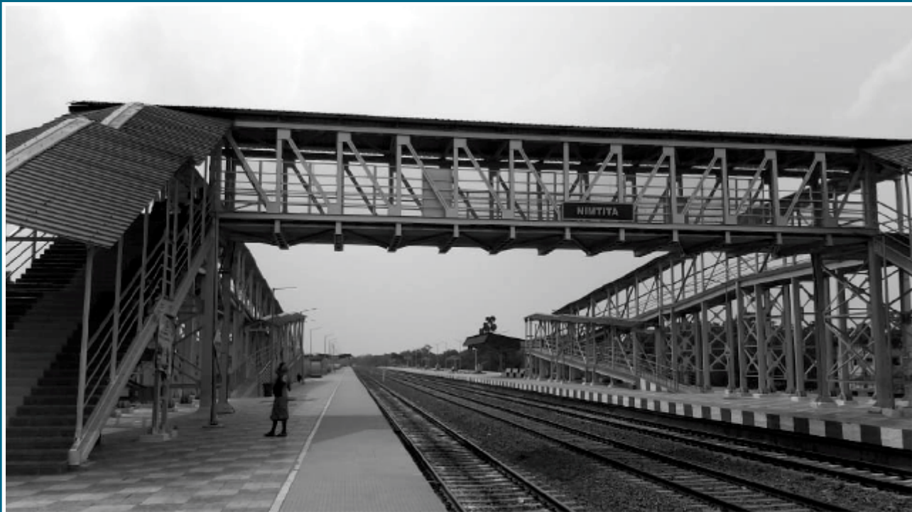
Laying of 19 KM Railway Track along with all the associated work like Platform , FOB , Building etc. in the section from Nimtita to Sujnipara for Eastern Railway
