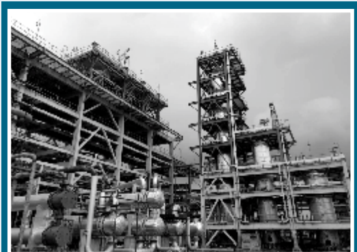
Civil, Structural and UG Piping works for New Process Units at IOCL Gujarat Refinery at Vadodara BS VI Project
